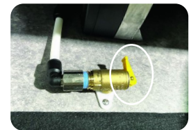
DRAIN VALVE- CLOSED POSITION FIGURE B
