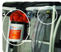
PUMP & 3-WAY VALVE FIGURE C
