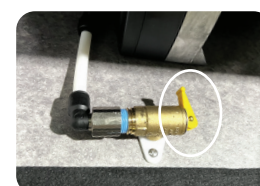
DRAIN VALVE- CLOSED POSITION FIGURE B
